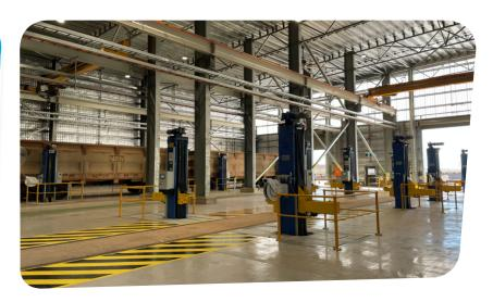
Coastal Electrics completed the E&I package associated with extending the RSM Workshop this included the installation of 2 jack systems, LV cabling, ELV cabling & communications cabling. Along with commissioning support for the OEM & FMG.
