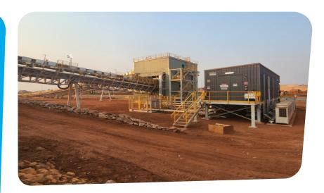
Coastal Electrics installed all LV, HV and communications cabling to the Stock Yard 2 Conveyor system inclusive of all switch room, transformer and field enclosure terminations. The site team completed all phases of testing prior to providing assistance to the client for commissioning.
