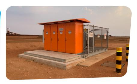
Coastal Electrics Installed 1.5km of 22kV HV cabling and fibre optic cabling from the Concentrate Handling Facility (CHF) to the Concentrate Diversion Pond (CDP), this included the installation and commissioning of one HV transformer, Kiosk Substation, multiple field instruments and pumps.
